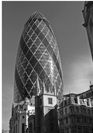
Figure 2 You can see the frame structure that supports this building.
